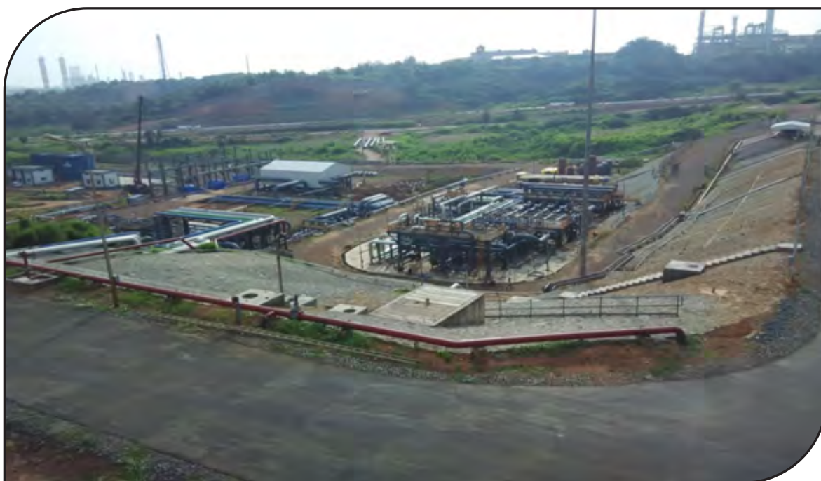
View of the aboveground facilities at Mangalore
