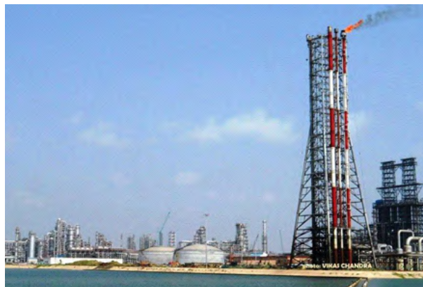
Diesel Hydrotreater Unit (DHDT)
