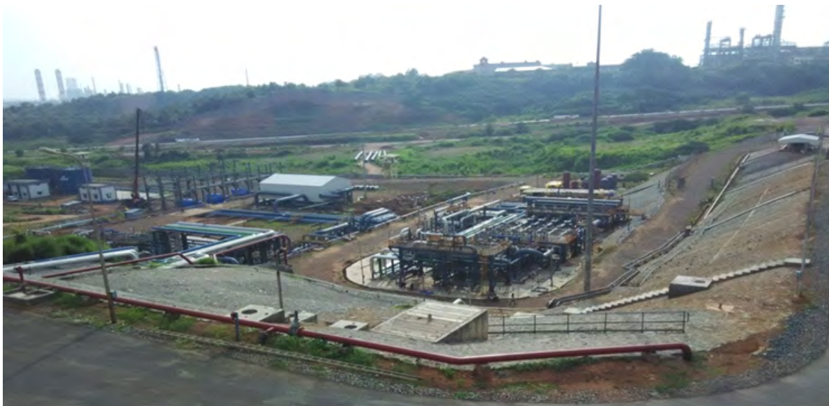
View of the above ground facilities at Mangalore
