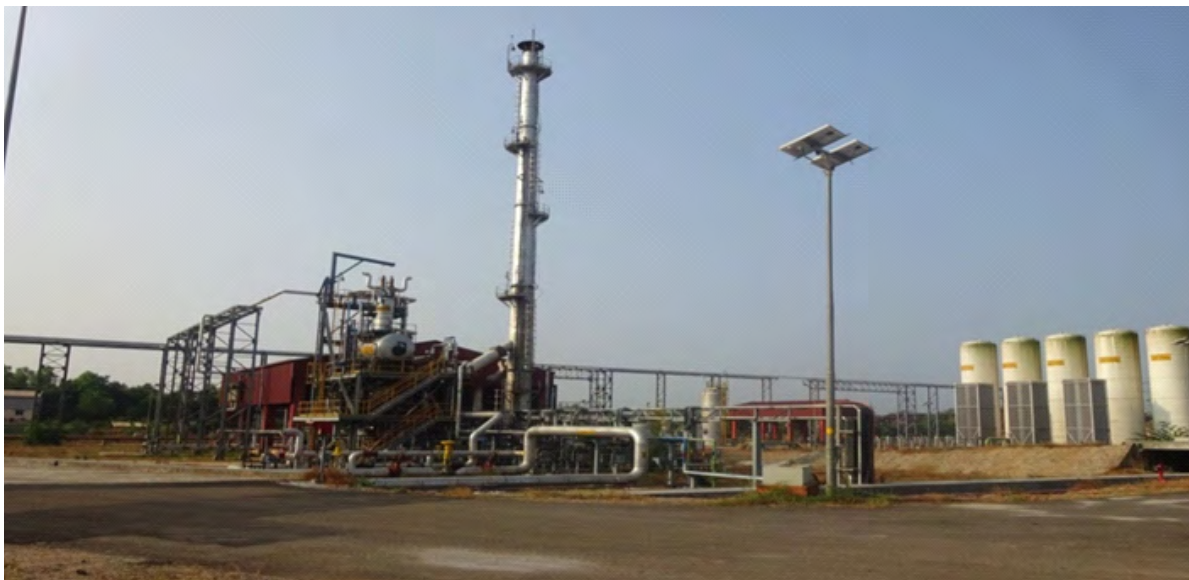
View of the above ground facilities at Padur
